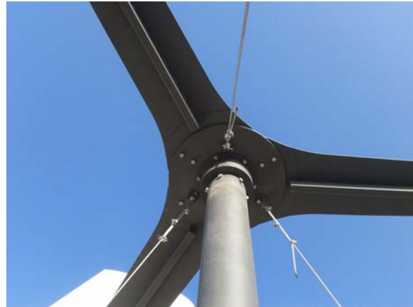
Figure 3: Upper Guy Wire Connection
