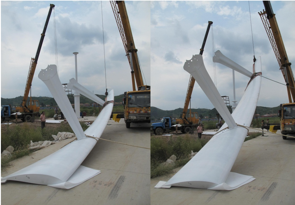
Figure 2: Lifting connecting arms and blades
